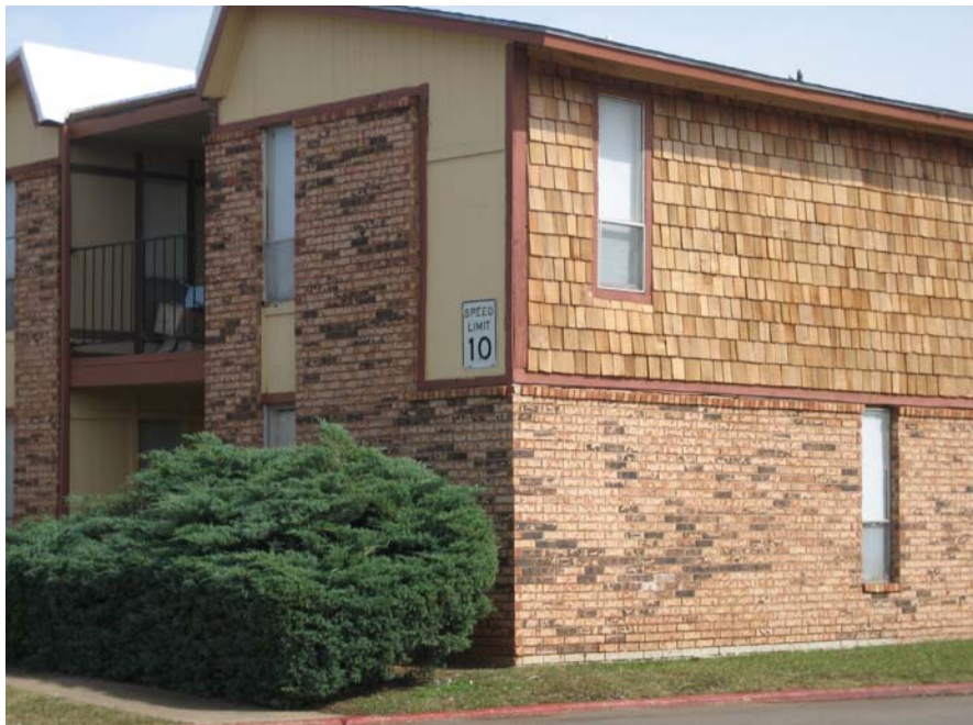
Example of Cedar Shingles which are currently being replaced on the entire property.
